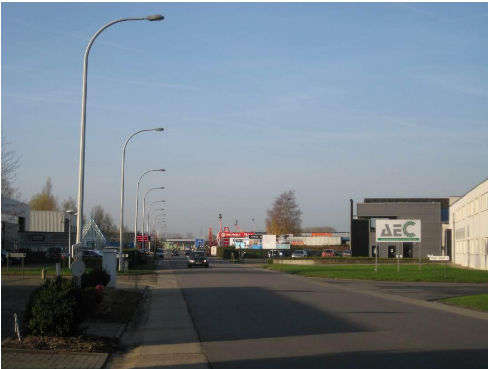
Image 1: Industrial area Nieuwland, new luminaires
