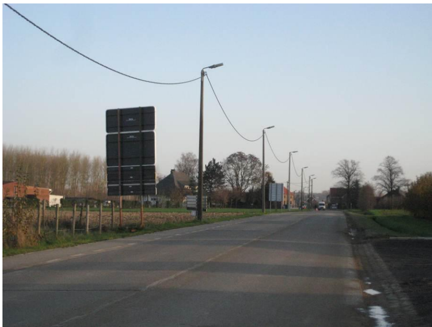
Image 11: Hoeledensebaan, existing lighting scheme
