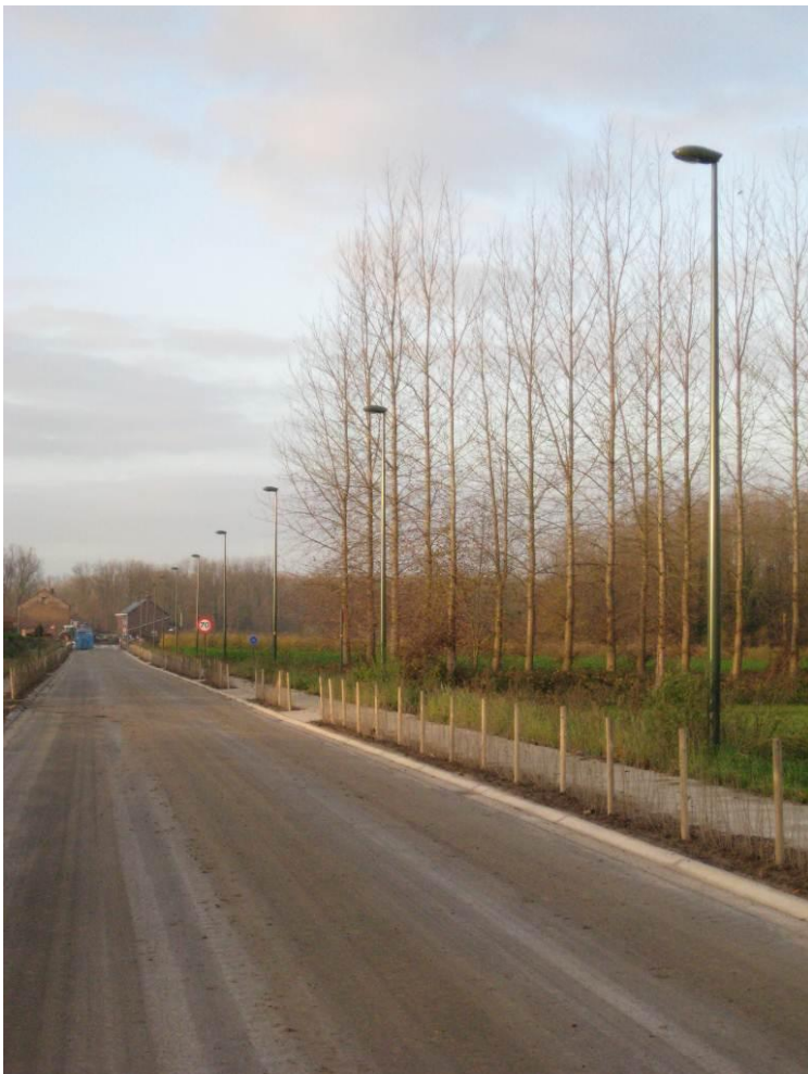
Image 13: Hoeledensebaan, new lighting scheme
