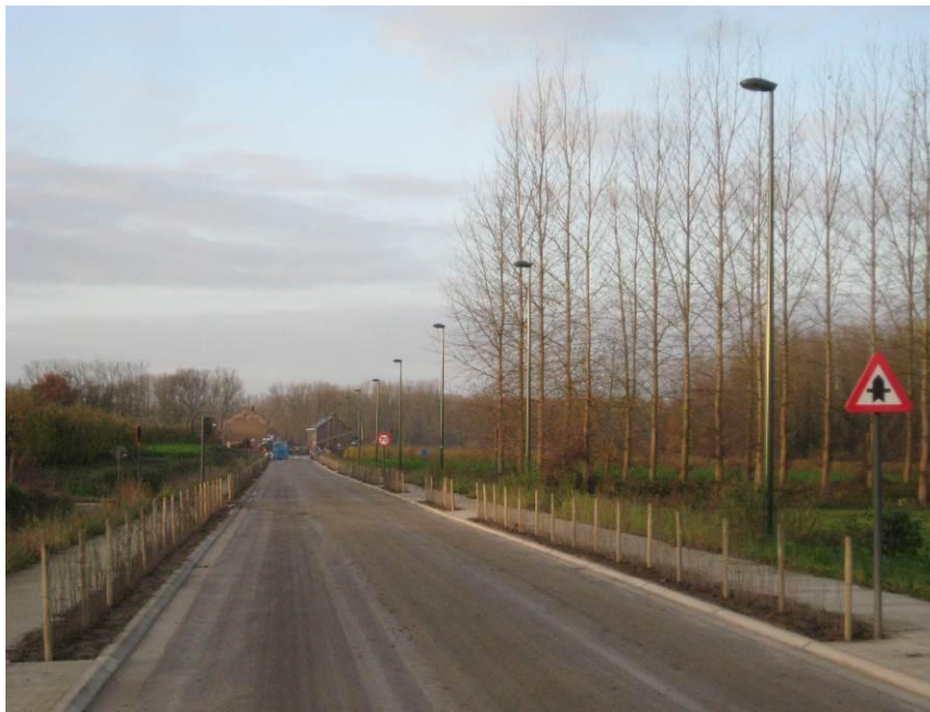
Image 1: Hoeledensebaan, new lighting scheme
