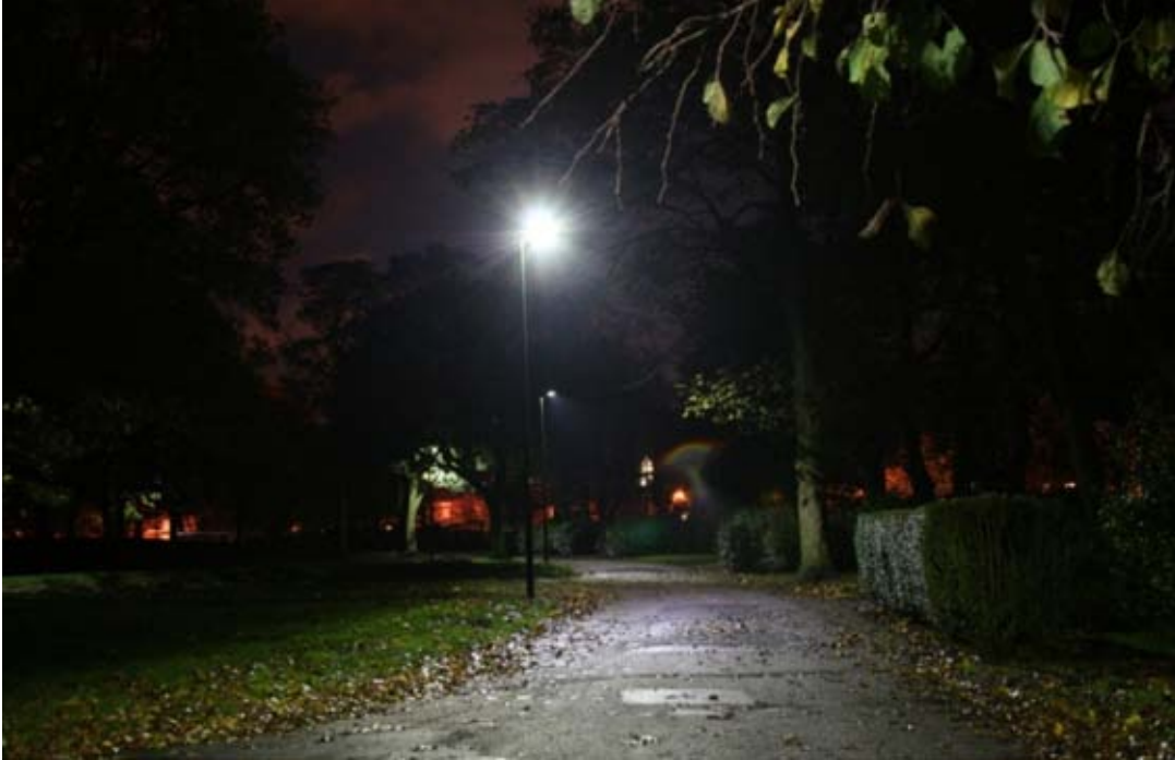
Introducing lighting into a heritage park brings economic and social value but uses energy, Victoria Park, St. Helens. (TCS 5.4)
