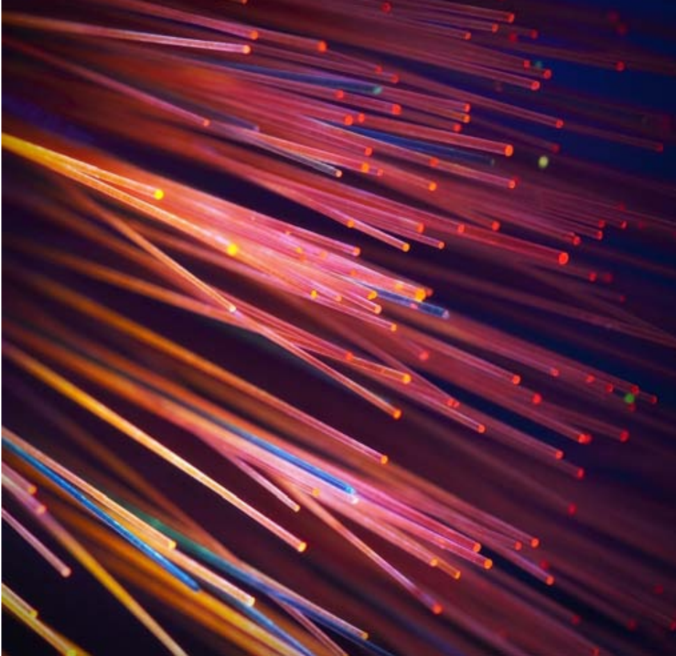
Fibre optic backbone installed at Strijp-S as part of the living lab for light innovation (TCS 6.1)
