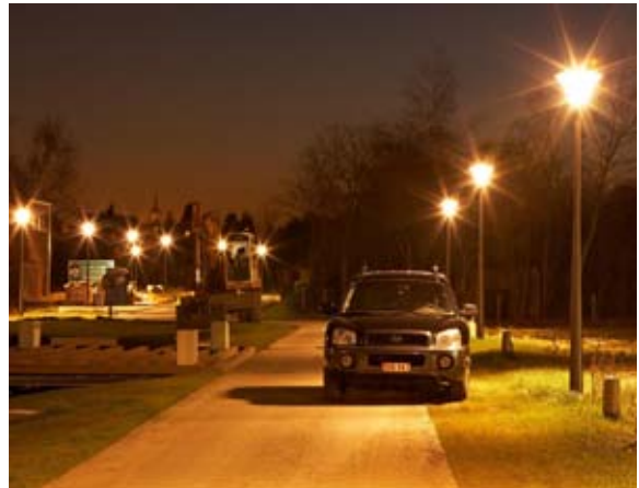
New white light Cosmopolis 60W lamp providing high-quality colour rendition and illumination compared to SON light source in surrounding residential areas. St. Helens. (TCS 7.1)
