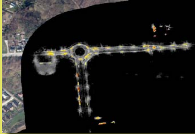
Excessive lighting levels can be identified using specialist aerial photography. St. Helens. (TCS 8.3)
